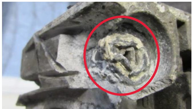
Damaged or broken device
