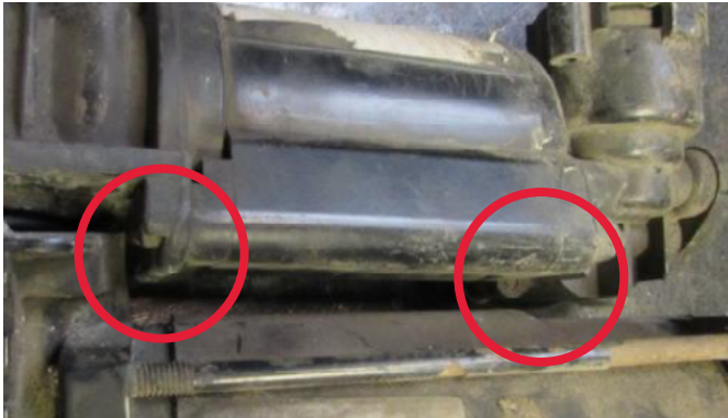
Device is dismantled
