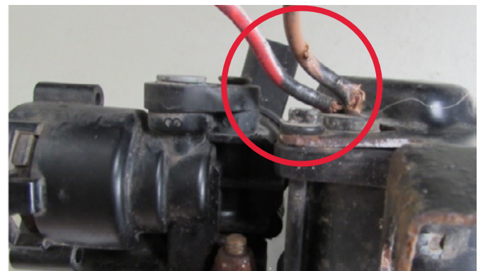
Cables shorter than 2 cm. Cables / wires damaged closer than 2 cm from housing.
